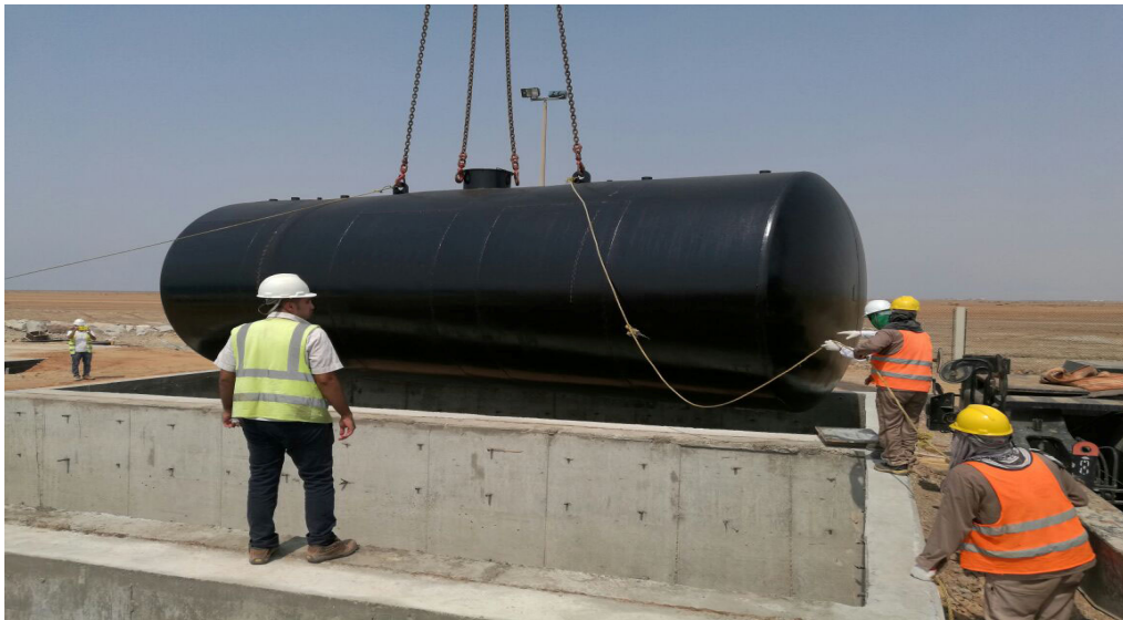
-Shoaiba ro phase 2 desalination plant fuel tank installation
